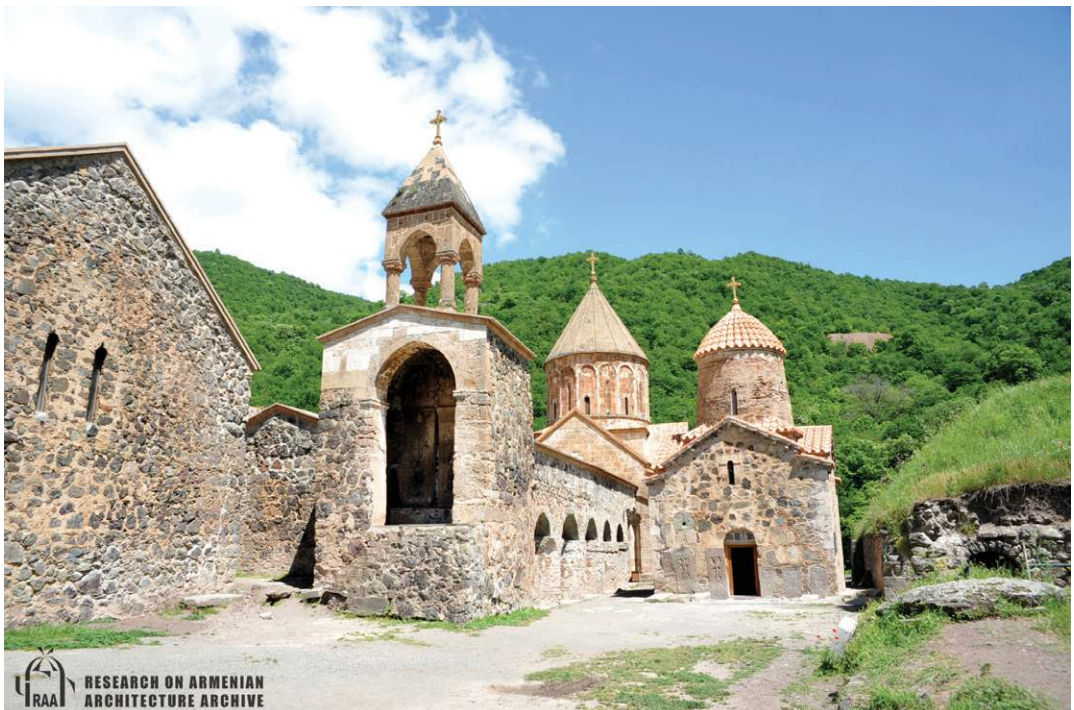
Figure 2. Dadivank Monastery in Artsakh (Source: Research On Armenian Architecture Archive)
