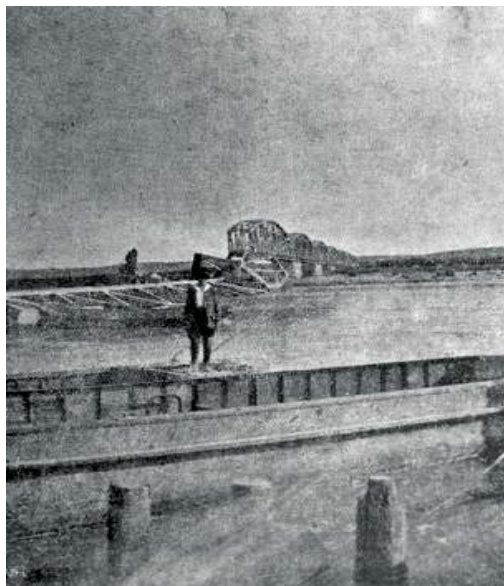
Figure 4. Railroad bridge across the Euphrates River near the Jarabulus station of Bagdad railway; it was partially destroyed by the explosives during the World War. The man in the photograph is Hansa himself.
